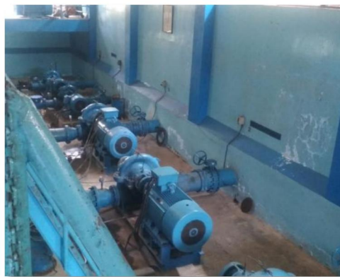
Gambar 18. Pompa Distribusi
